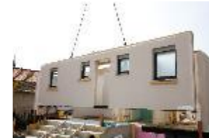
Transforming construction (up to £170m)
